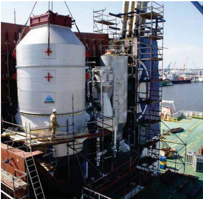
Fig.: Scrubber system arrangement.
