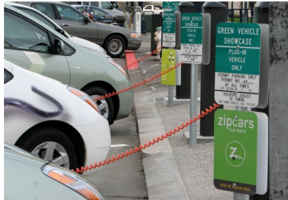
Fig. Infrastructure for Plug-In Vehicles in San Francisco
