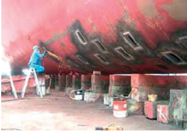
Fig: WAIP installation process in dry dock
