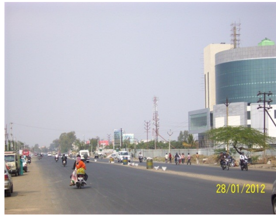
Figure-3 No Street lighting and markings
