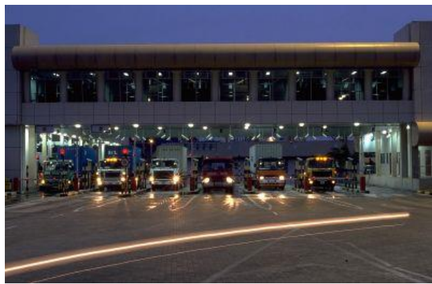
Fig 2.Flow through Gate (Singapore Port)
