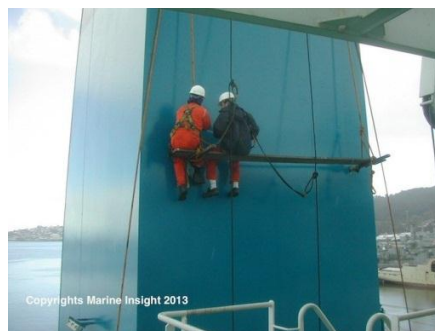
Figure 3.1.1 Working at heights
